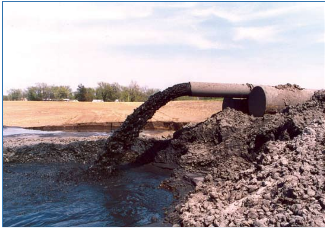
Dredging slurry exits the pipe at the settling basin.
