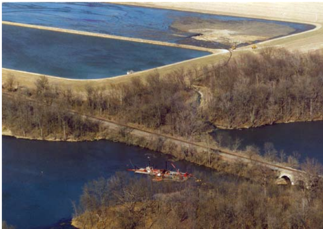
A hydraulic dredge pumps material to a settling basin (top right).
